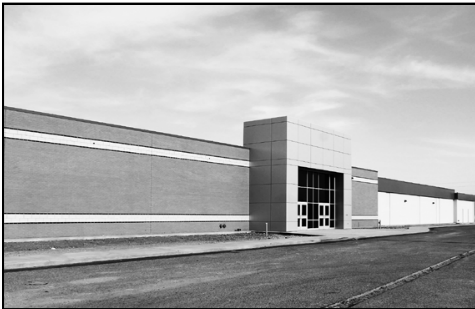
The new Lubbock Center, still under construction on April 26, is expected to be ready for the fall semester.
